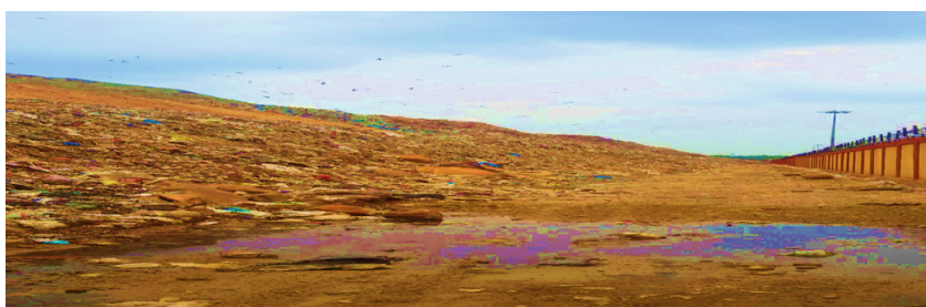
Fig. 3: Okhla Landfill Leachate (backside view) Source: Sonam
