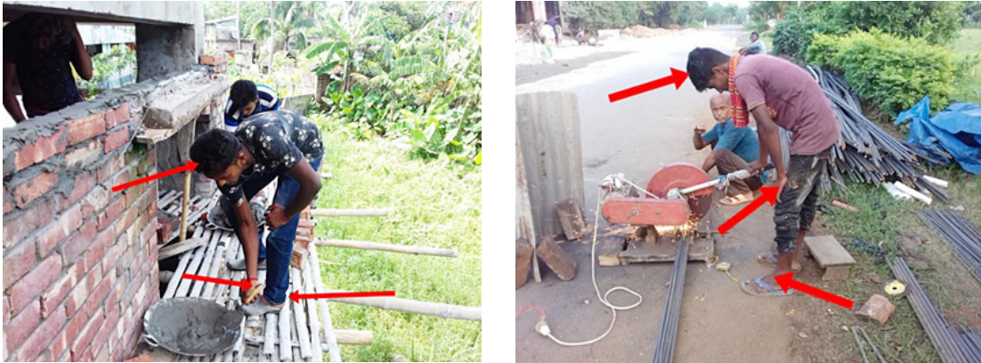
Fig. 7: Ironwork and bricklaying tasks
