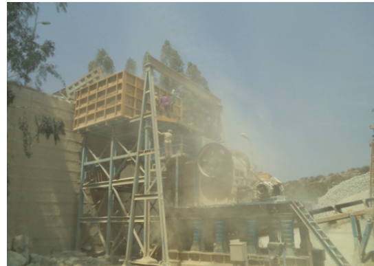
Fig. 6: Lack of dust suppression measures in primary hopper area
