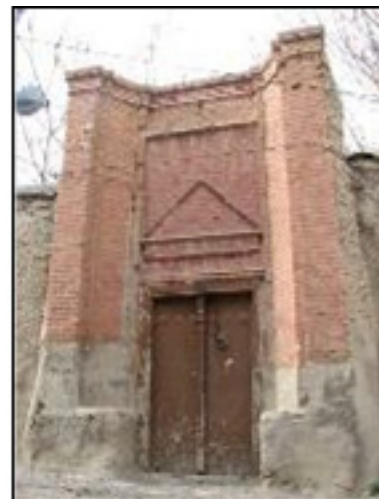
Fig. 14: The house entrance Of Qajar era near Jeme mosque, Authors
