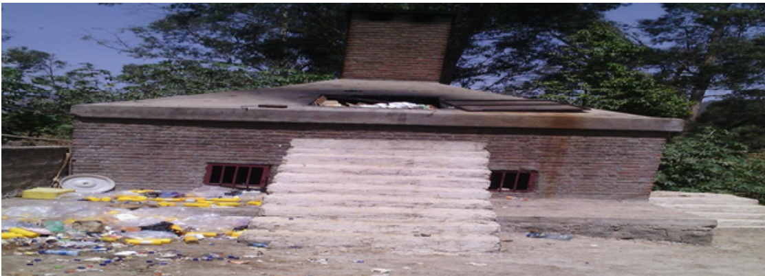
Fig. 5: A newly built incinerator for HCW incineration of Menellik II Hospital, February 2015
