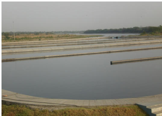
Fig. 4 (a): View of UASB Reactors (b) Final Polishing Ponds
