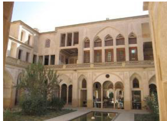
Fig. 7: Shading with tall walls surrounding the central courtyard (Abbasid House in Kashan, writer, 2012)
