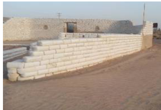
Fig. 9: The use of sand bags for building construction (Maranjab are) (writer, 2014)
