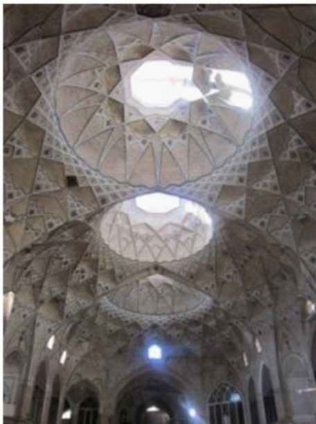
Fig. 18: Application of Yazdi bandi with a geometric structure for creating a clear and colorful atmosphere: authors
