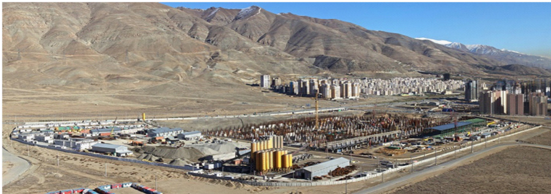
Fig. 1: Case Study project overview
