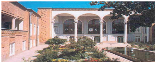
Fig. 2: The house of “Qadaky” One of the best samples of traditional architecture (Haeri et al., 2008)
