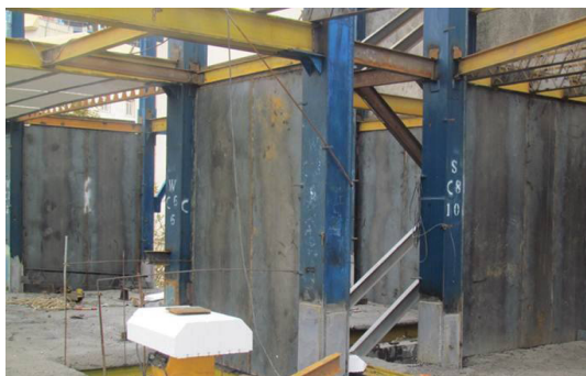
Fig. 1: Left: performed steel shear wall. Right: schematic figure of steel shear walls (with or without Stiffeners)
