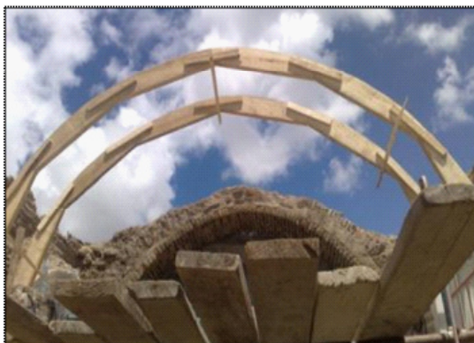
Fig. 7: Wooden template implementation as tavizeh – Shami Caravansary- Zanzan.
