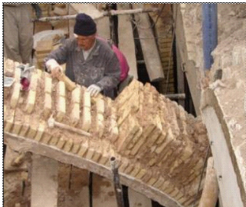
Fig. 15: Implementation of the wing and the body of tavizeh.
