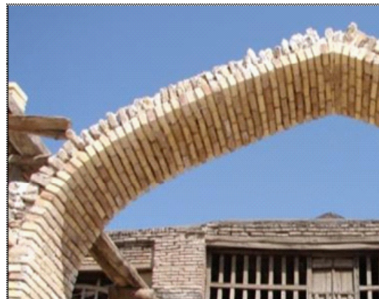
Fig. 14: Decorative bricklaying implementation on the wing of tavizeh.
