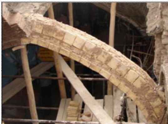
Fig. 11: An example of a tavizeh with Zarb bricklaying.
