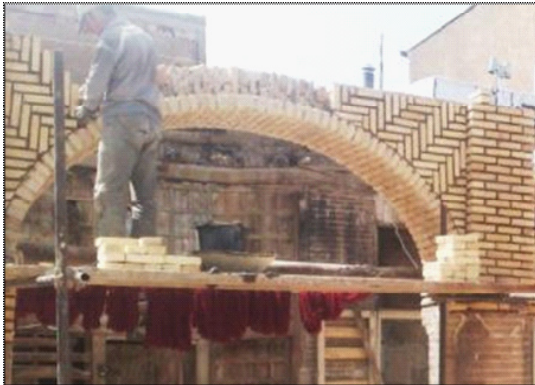
Fig. 19: Implementing decorative bricklaying on outer edge of the wing of tavizeh- Dokhan-Caravansary in Bazzar-Zanjan
