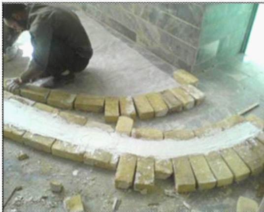
Fig. 5: A plaster tavizeh with Kalil-chafd that is prepared and dried on the flat ground.
