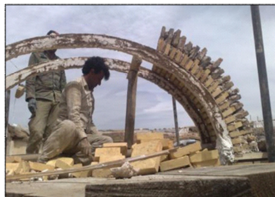
Fig. 8: Assembly of two pieces of plaster templates in Herreh tavizeh. Shami -Caravansary, Zanzan.
