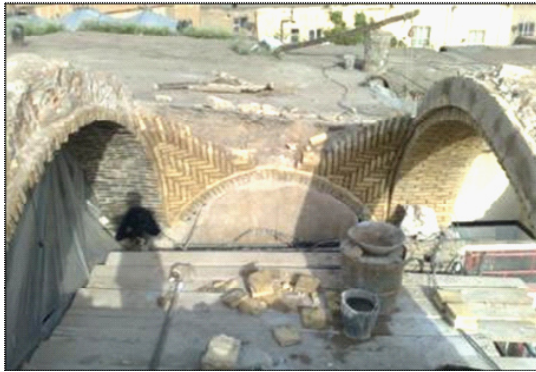
Fig. 17: Implementing Kajaveh arch on the inner edge of the wing of tavizeh- shami-Caravansary, Zanjan.
