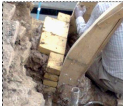
Fig. 16: Placement of bricks in the wing and the body of tavizeh.
