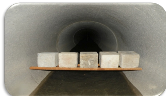
Fig. 7: Arrangement of the samples in the empty space above the sewers.
