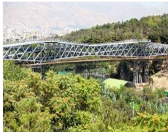
Fig. 3: Nature bridge, Tehran
