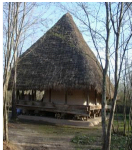
Fig. 5: The scape of a rural house in mild and humid climate
