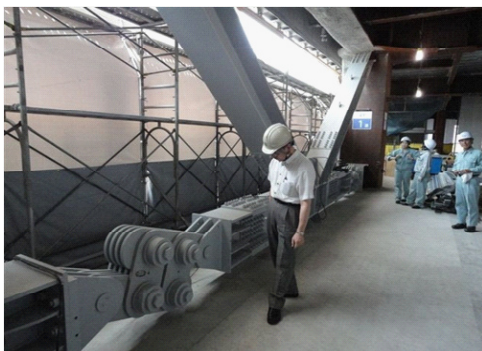
Fig. 10: Friction dampers
