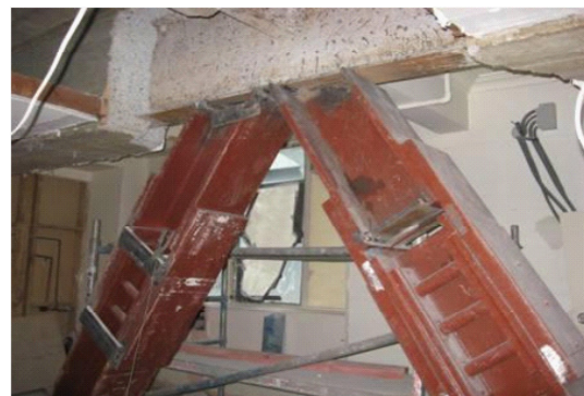
Fig. 11:Yielding damper(Steel brace)
