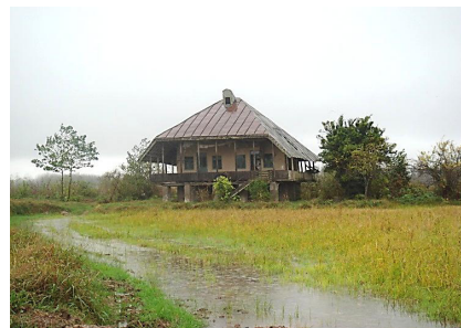
Fig. 2: Formation of a semi-enclosed space around a central enclosed space, Estakhr-e Bijar village near Astaneh Ashrafieh, (source: authors)
