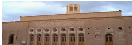
Fig. 22: To stay summer room, door the room on the west side
