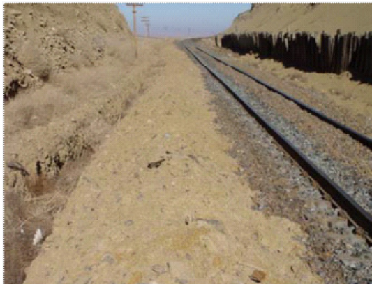
Fig. 5: Sides improper drainage line
