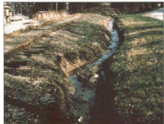
Fig. 5: Sides improper drainage line
