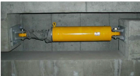
Fig. 17: installing viscous dampers on the floor and foundation in structures
