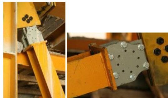
Fig. 5: The place of PVD damping installation
