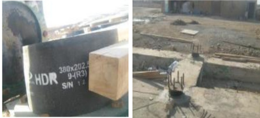
Fig. 21: using HDRB damper in Ray-Iran
