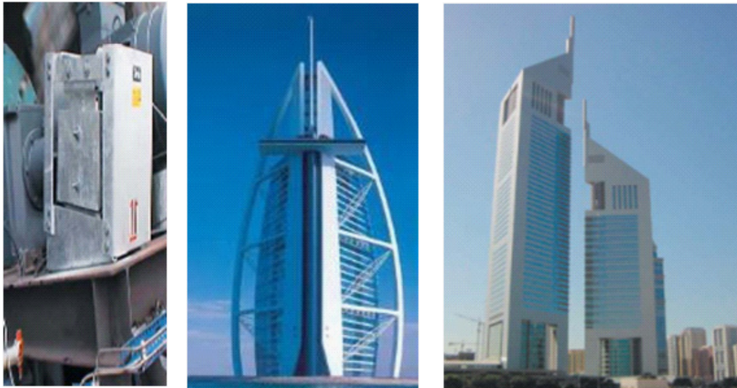
Fig. 25: using a TMD damper in towers of Dubai
