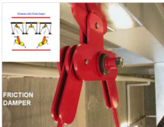
Fig. 4: Using rotational friction dampers in retrofitting[5]
