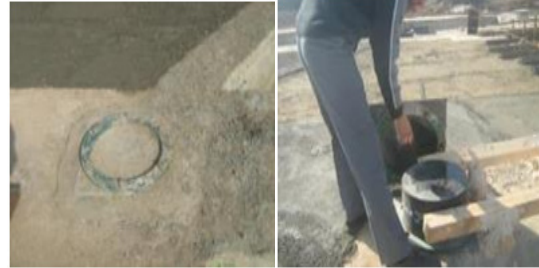
Fig. 22: HDRB damper installation to dealing with uplift
