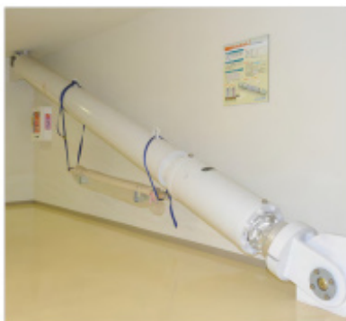
Fig. 15: A view of viscous damper
